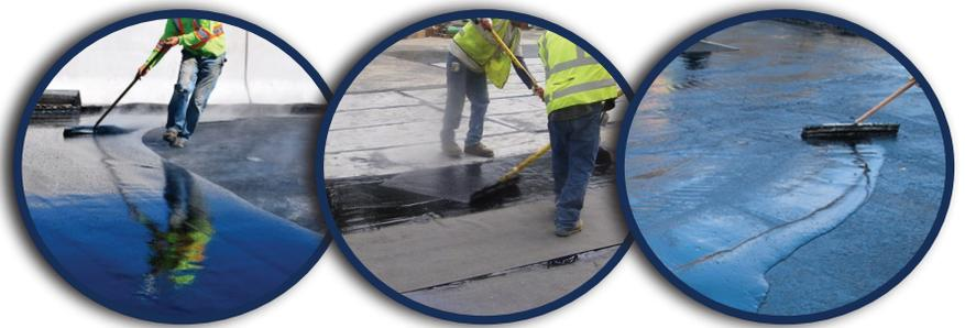
**RamTough 250 is a hot applied rubberized asphalt membrane** which forms a completely monolithic, waterproof system without seams or joints.
