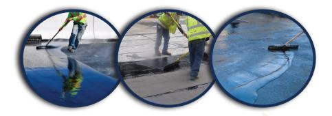
**RamTough 250 is a hot applied rubberized asphalt membrane** which forms a completely monolithic, waterproof system without seams or joints.
