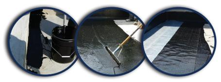
**Black Pearl is a unique COLD fluid waterproofing system** designed to go on green and damp concrete along with being installed at temperatures that commonly are not allowed by other technical platforms.
