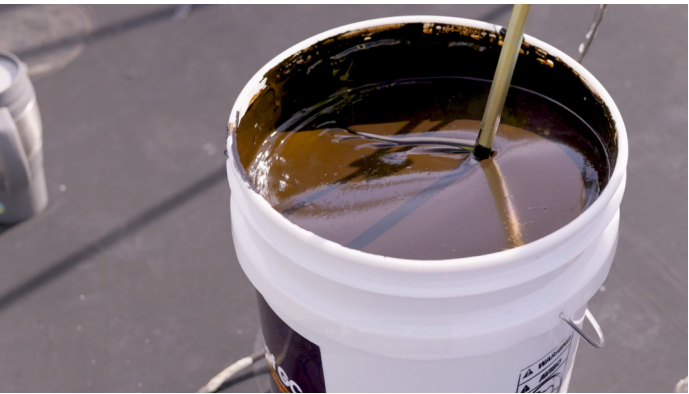
PICTURED: Contractor uses a mechanical mixer to slowly mix the RamProof GC material before it is applied over the substrate. Mixing the material at a slow speed helps to prevent bubbles or air pockets.
