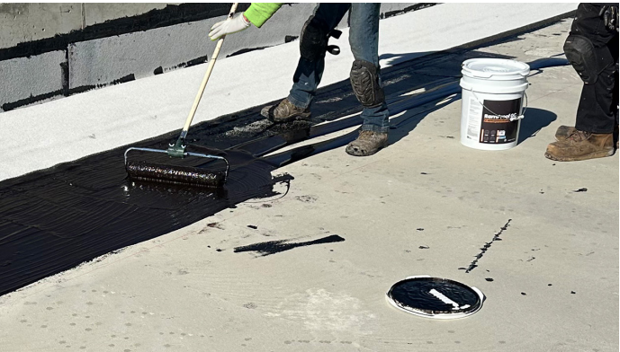
PICTURED: RamProof GC applied evenly across a concrete surface with a roller. RamProof GC is available in multiple grades including squeegee, roller, spray, and trowel-grade, depending on the project.
