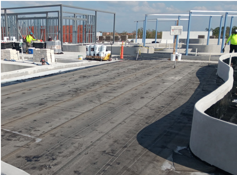
PICTURED: RamProof GC is reinforced with Barrett Ram 203 fiberglass-reinforced SBS-modified asphalt protection course, followed by a layer of approved drainage material and a concrete topping slab over the entire assembly.
